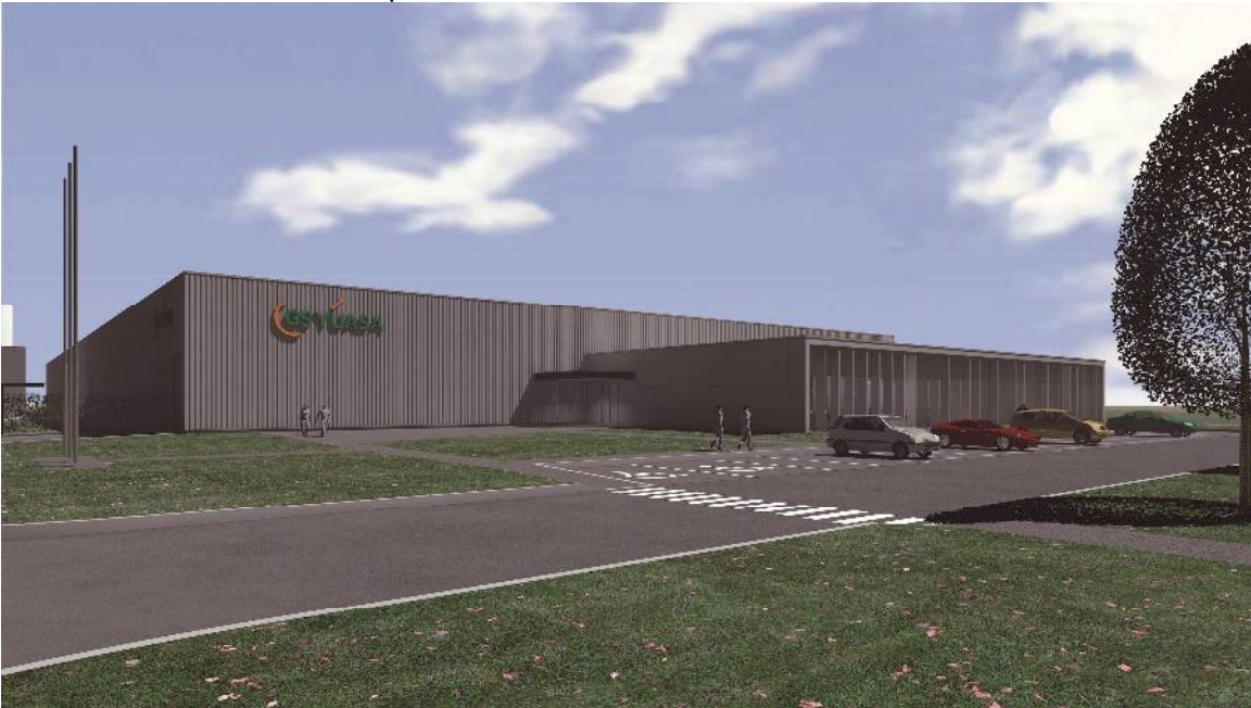
1. External view of the new plant
